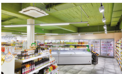
Retail Commercial refrigeration
